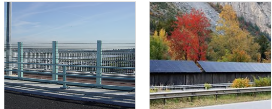
Figure 14. Clear Acrylic and Photovoltaic Noise Barrier Examples (Gramm Barrier Systems Fanzun, Architects and Engineers)
