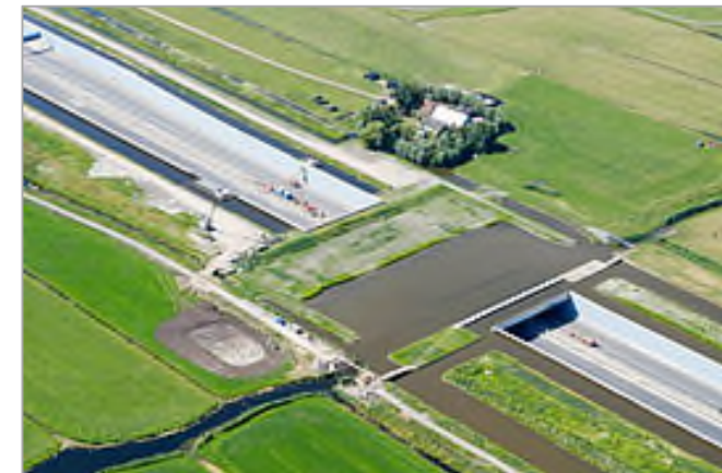
Figure 10. ‘Eco-aqueduct’ over ‘sunken’ motorway on the new A4 in Holland (Google)
