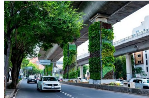
Figure 12. Overbridges Example (New Civil Engineer)
