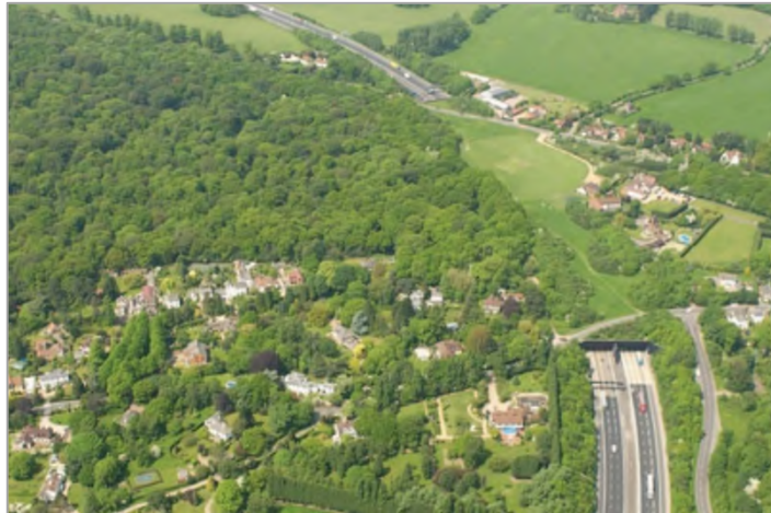
Figure 8. M25 Bell Common Tunnel – Costain (CIHT Award for Major Projects)
